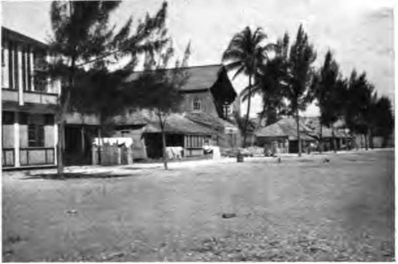
PORT ROYAL. End of Chapel wrecked by Earthquake.
